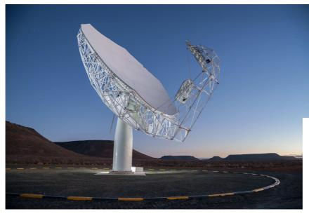
The first of the planned 64 MeerKAT antennas erected outside Carnarvon, Northern Cape. The dish has a diameter of 13.5 m while the total structure is 19.5 m high and weighs 42 tons. (Credit: SKA South Africa, www.ska.ac.za)
